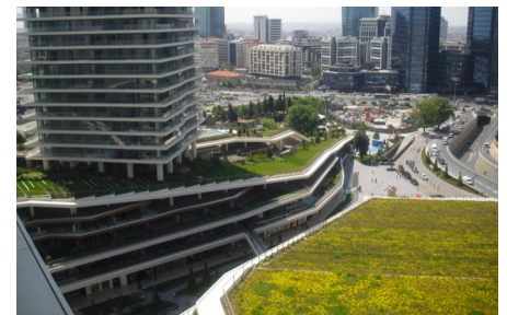
The intensive green areas with their shrubs and trees as well as the paved zones of the courtyard were all realized based on the Floradrain® FD 40-E drainage element, whereas the extensive green roof of the theatre is based on Floradrain® FD 25-E.
